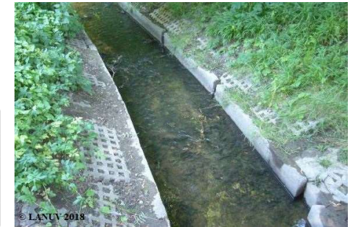
Bed made of concrete / grid stones with sediment
