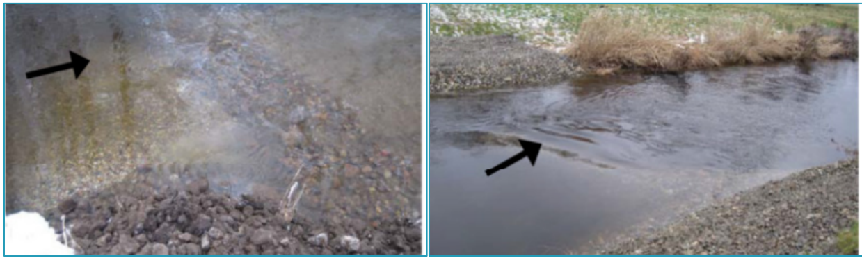
Figure 14: Gravel micro-groin and bank protection made of coarse gravel and cobbles, with finer gravel piled upstream as a spawning substrate (left); gravel micro-groin with bank protection on both sides (right); Photos: L. Tent
