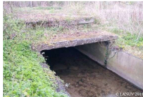
Piping of a stream with sediment.
