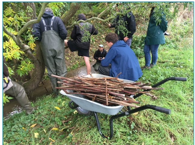
Figure 7: sedimented stream section (top), installation of hazel rods as wood structures (bottom) © Benjamin Gottfried
