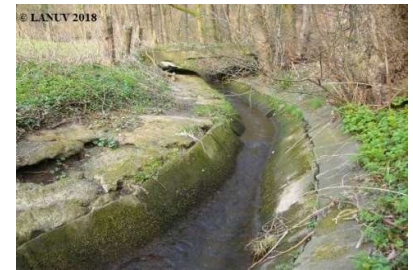
Dilapidated bank shoring with wooden planks (above) and solid bank shoring with concrete slabs (below).
