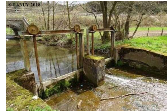
Technical backwater caused by a transverse structure. Natural backwater is caused, for example, by wood accumulations or beaver dams.
