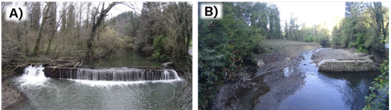
Figure 10: Before (A) and after (B) of the removal of one of 8 dams in the Deba river, Spain. This restoration helped restore 28km of free flow to the river.
